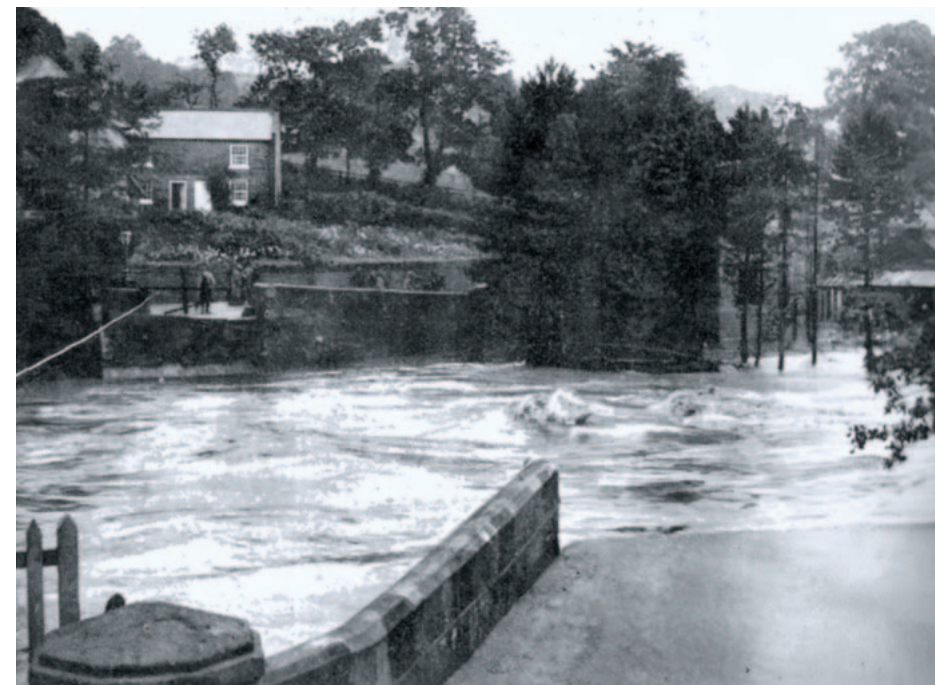
Bridge over the Esk at Sleights swept away.
