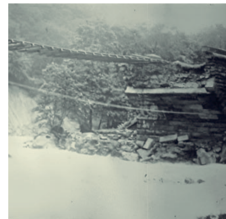
Wrecked railway bridge at Glaisdale, 1930s flooding.
