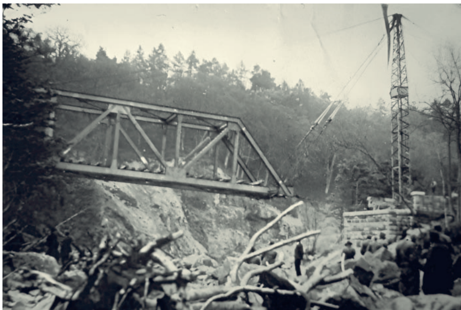
Replacing the wrecked railway bridge at Glaisdale, 1930s flooding.
