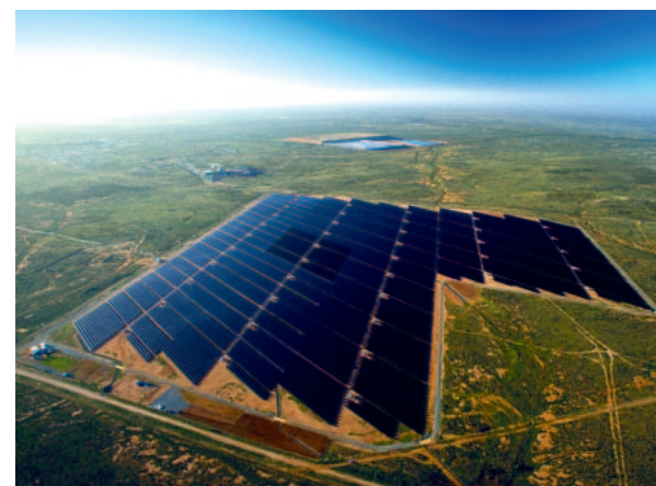
Solar power in Australia.
